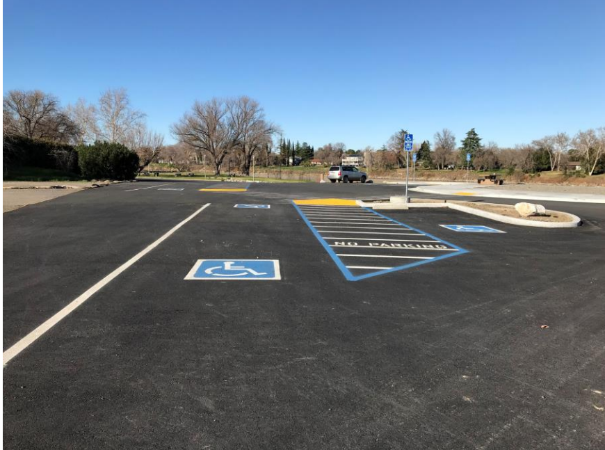
ADA parking, curbs, and sidewalk at the boater parking area
