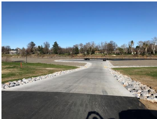
Access roadway from the parking area to the boat ramp
