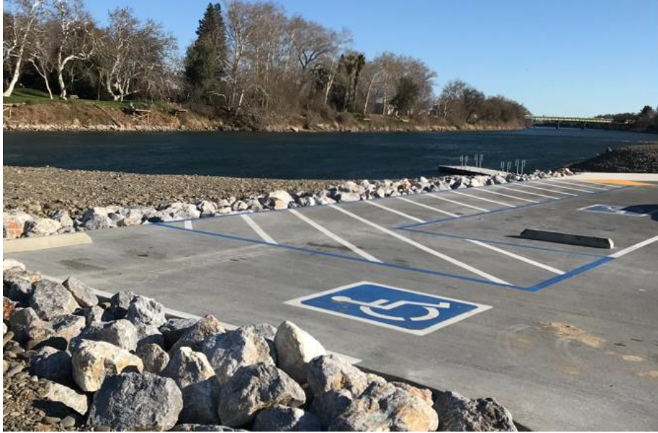
ADA parking and riprap near the top of the boat launch ramp
